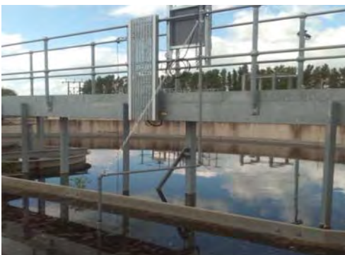
Final Settling Tank
