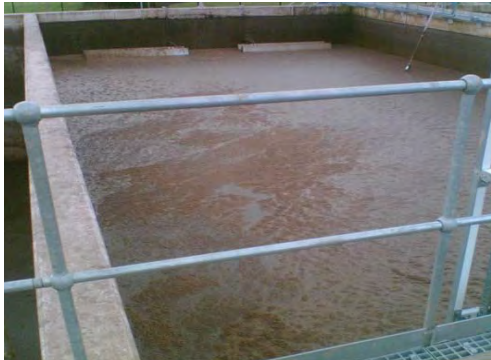
Sequencing Batch Reactor (SBR) Tanks
