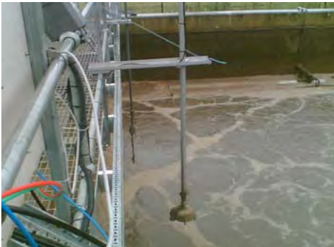
Sequencing Batch Reactor (SBR) Tanks
